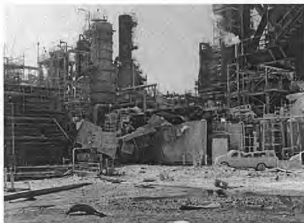
The 2015 ExxonMobil Torrance explosion helped spur proposed PSM reforms.
